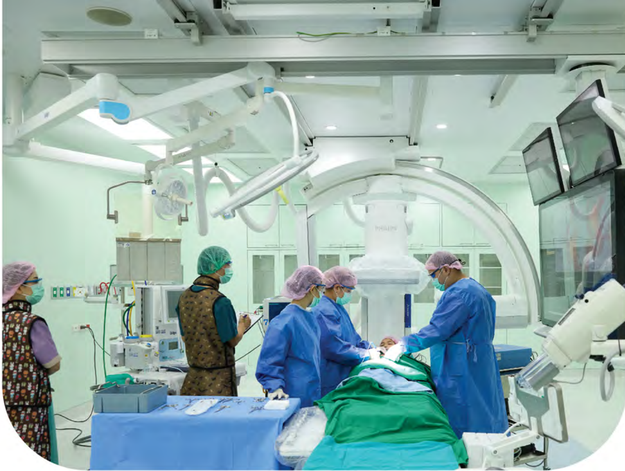
Equipped for immediate response, the hybrid operating room enables X-ray imaging without transferring the patient.
